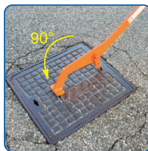
● 90° rotation of the key and hooking of the slot
